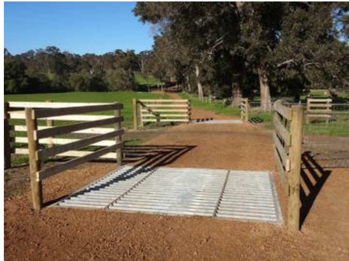
Stock grids along rail trails, such as this one on the newly opened extension of the rail trail south of Margaret River in WA, can allow stock crossings to be open 24/7 thereby enabling stock and machinery to cross the trail unimpeded.
