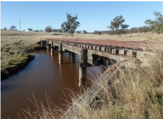
Repairing bridge abutments and installing decking and handrails will be essential tasks in making safe the numerous bridges along the proposed rail trail between Merriwa and Sandy Hollow.
