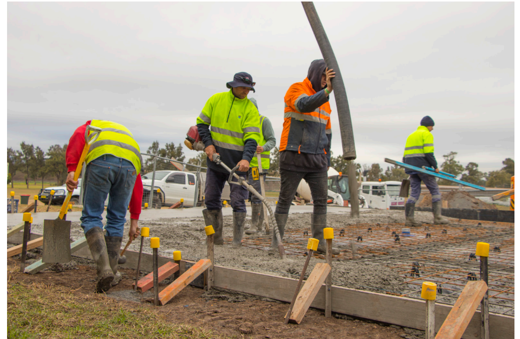
Concrete foundation being poured for the White Park canteen, July 2019
