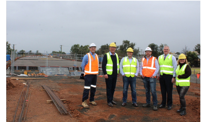
Scone Bypass under construction - July 2019
