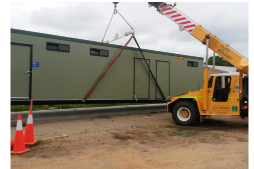
Merriwa Showground amenities block crane delivery March 2020
