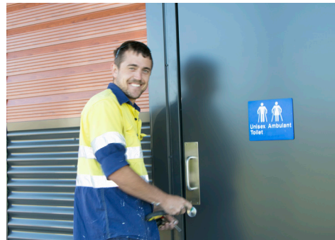
Amaroo Park in Scone toilet under construction, April 2020
