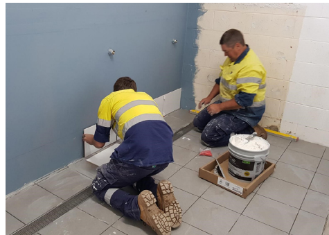
Council staff upgrade the Merriwa Oval 1 change-room, November 2019
