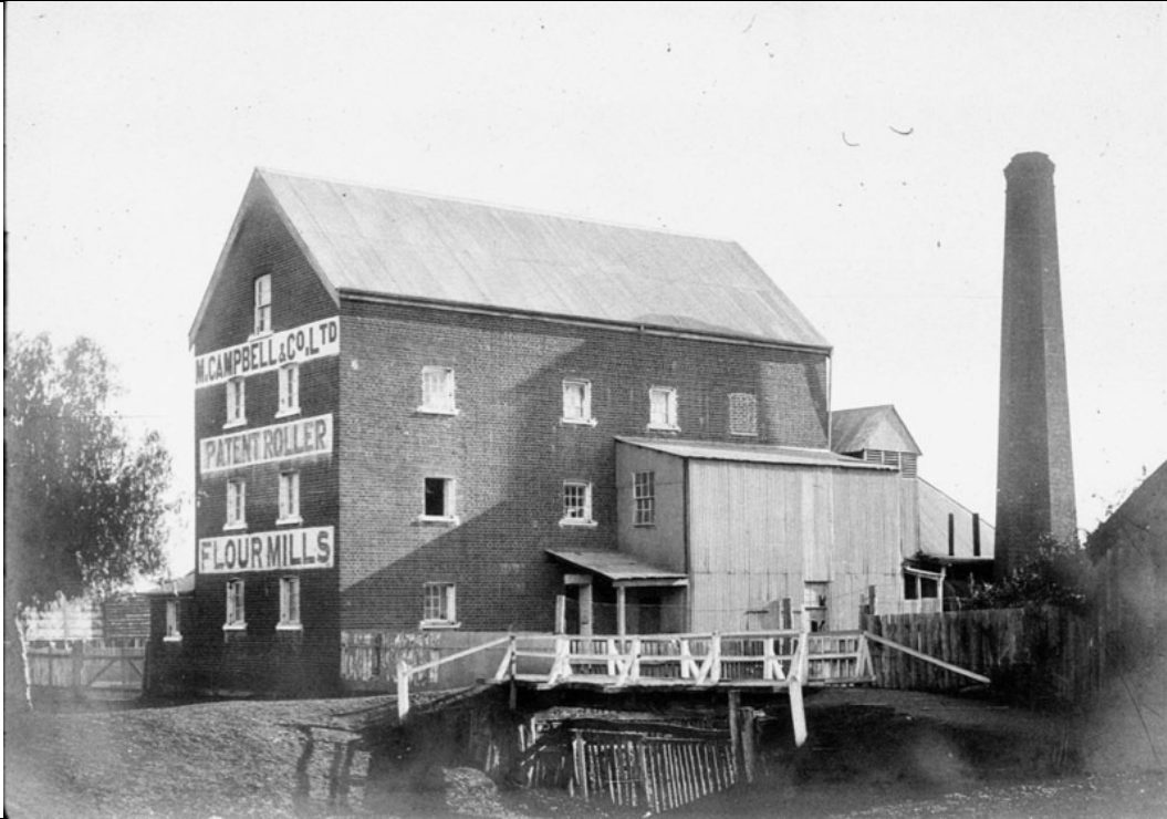
Figure 9: Campbell's large four mill in Guernsey Street at Scone c1910. This mill building survives as part of the Scone RSL club. (Source: SLNSW)
