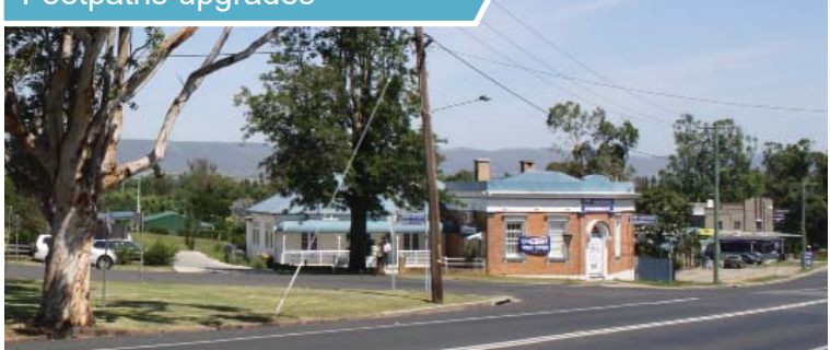
There is a lack of footpaths in the town core near the intersection of Segenhoe and Macqueen Street
