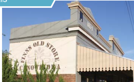
Painted facade, Canowindra NSW
