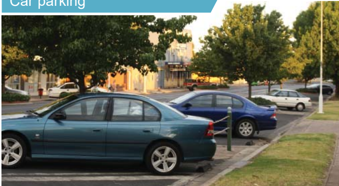
45° parking (rear to kerb) with rear wheel stops in Cowra NSW
