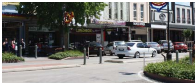
Landscaped blisters make it easier to cross the road in Goulburn, NSW
