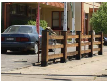
Fencing a driveway next to the footpath helps to separate cars and pedestrian. Murrurundi, NSW.
