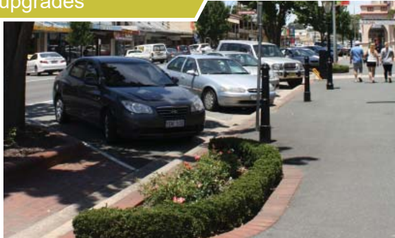
Asphalt footpath, with brink paving inserts in Yass, NSW
