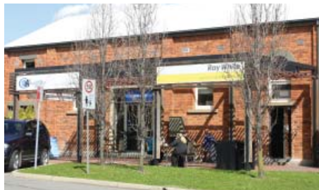
Existing outdoor seating on St. Aubins Street
