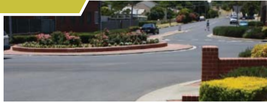
Example of a roundabout with low level landscaping in Yass, NSW.
