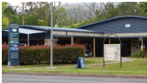
This shared facility at Murrurundi includes the tourist information centre, a cafe, Centrelink and a medical centre
