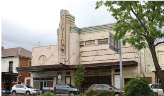
The Civic Theatre features could be highlighted with paint
