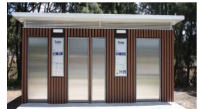
Self-cleaning public toilets, Mudgee NSW
