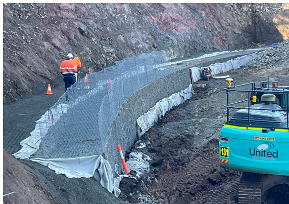
Gabion wall & Earthworks
