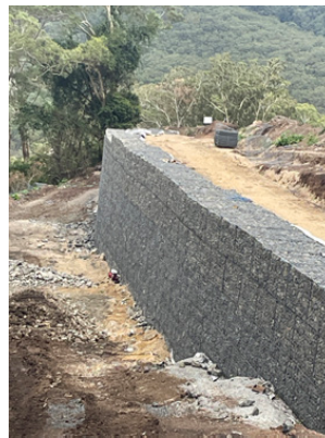
Section 3 Gabion Wall construction
