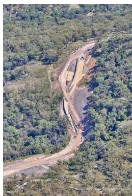
Section 3 Gabion Wall construction
