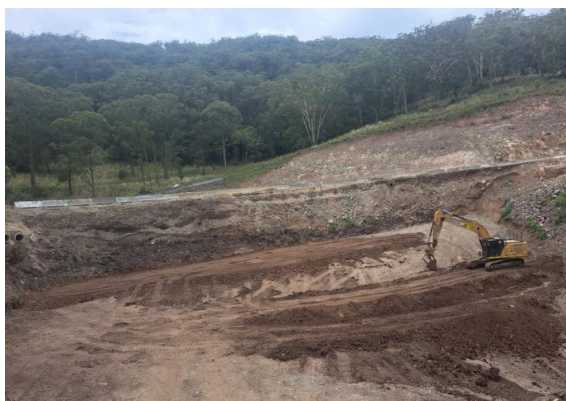
Section 2 Hairpin Excavation and backfill
