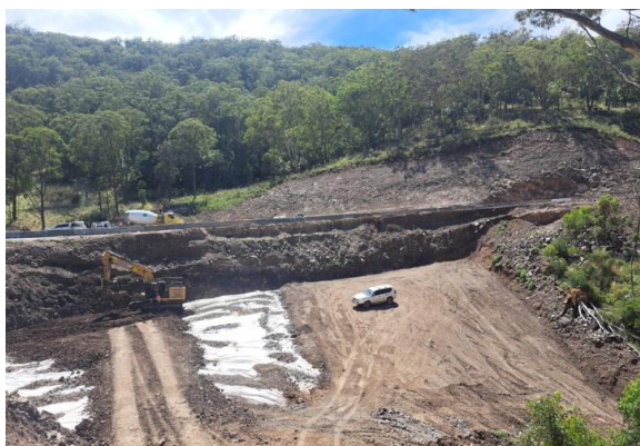
Earthworks Gabion wall construction
