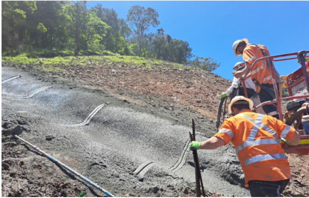
Shotcreting Stormwater Channel
