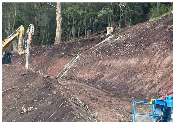
Rock Bolt Installation
