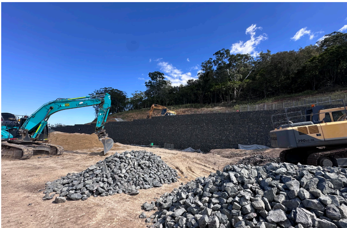
Completed Gabion Wall
