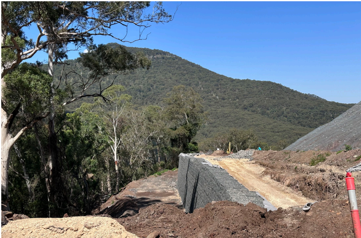
Completed Gabion Wall
