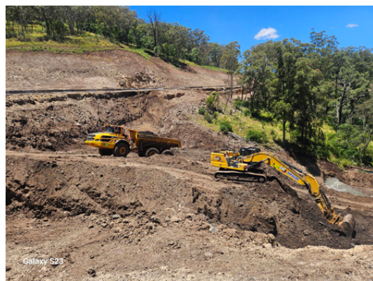
Section 2 Hairpin Excavation and backfill
