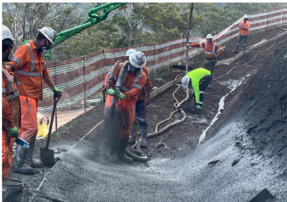
Catch Drain Shotcrete
