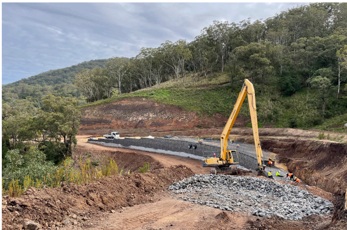
Gabion Wall Construction
