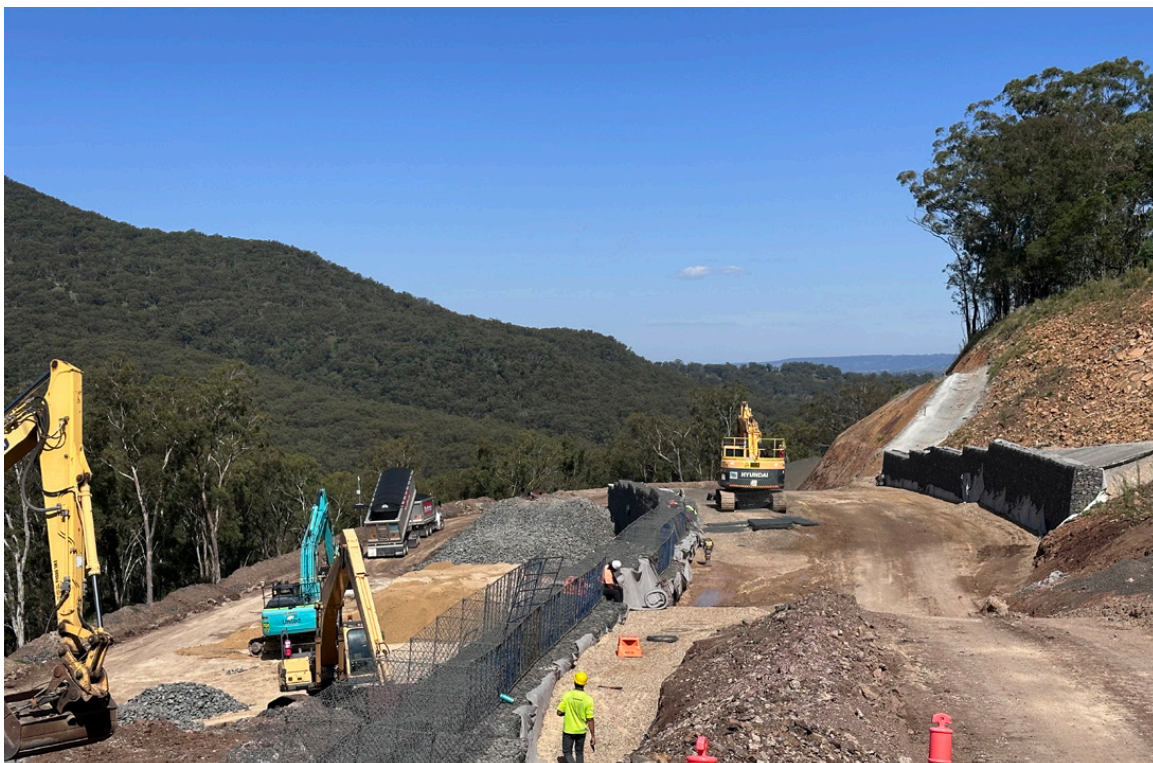
Pavement, Gabion Wall, Catch Drain.
