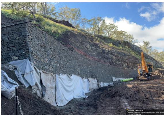
Gabion Wall Construction
