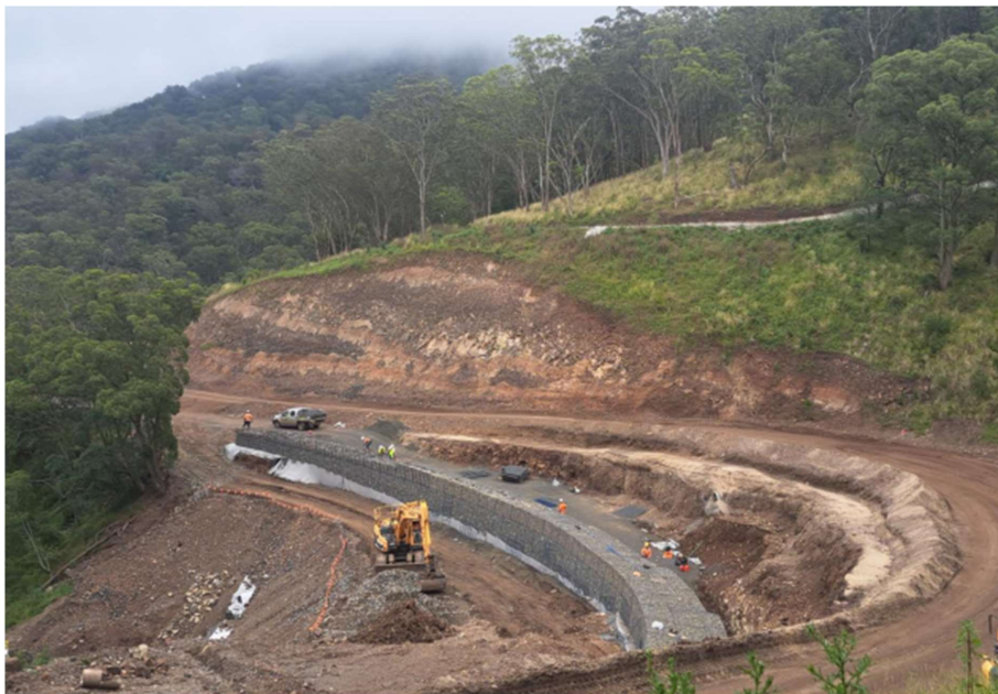
Gabion Wall Construction – Section 3
