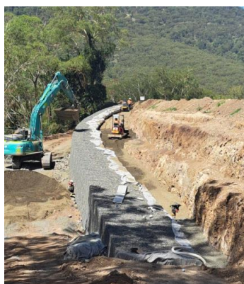
Section 2 Gabion Wall
