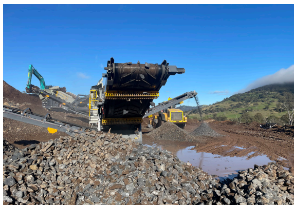
Manufacture Gabion Rock at TSR
