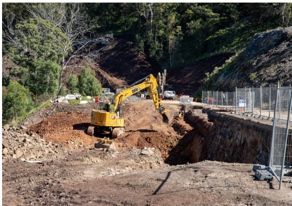
Excavations for gabion wall construction
