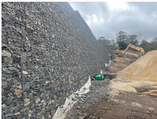
Section 3 Gabion Wall construction
