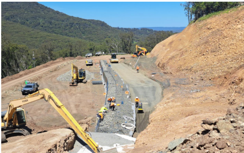
MT 60 Gabion Wall Construction - Level 8 Install & Backfill
