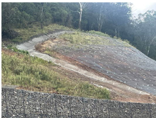
Section 3 Gabion Wall & Drainage Shute
