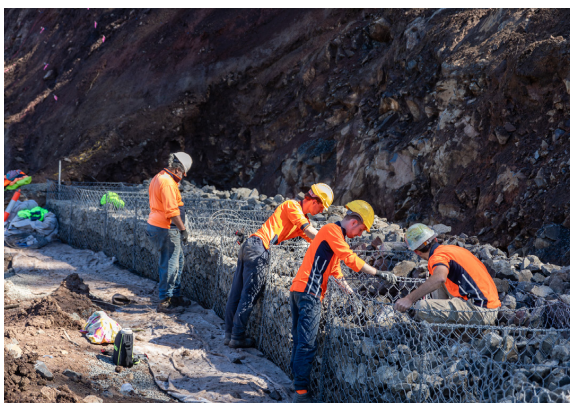
Gabion wall construction
