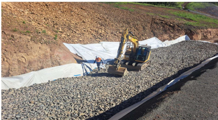
Drainage Blanket – Section 2
