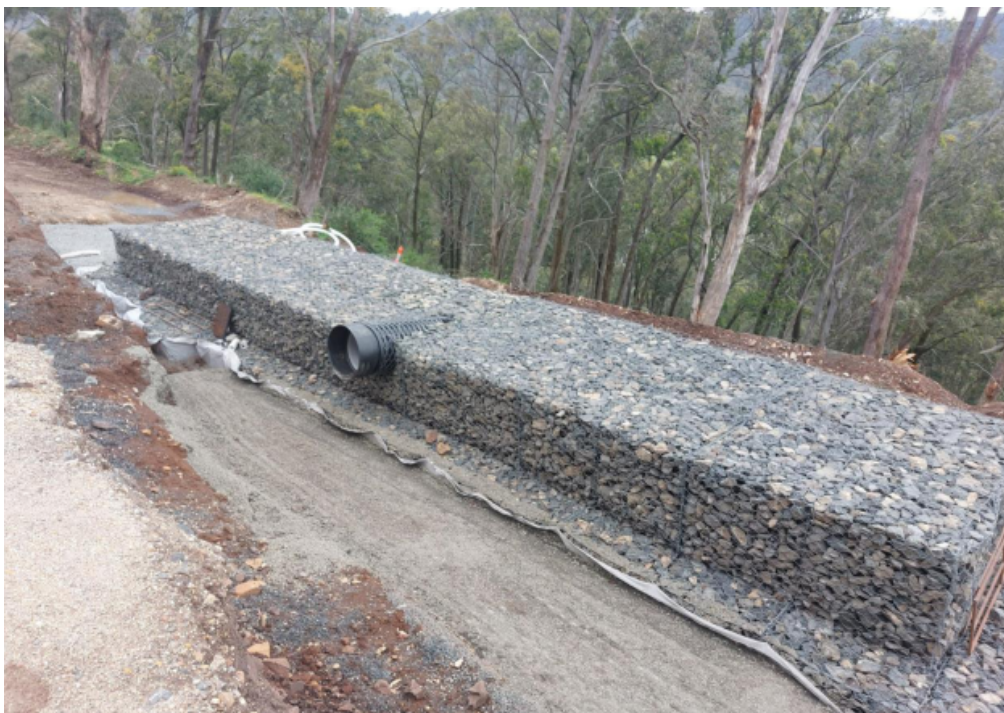
Stormwater Pipe Front & Rear Views
