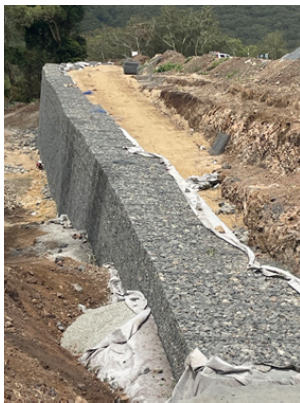
Section 3 Gabion Wall construction
