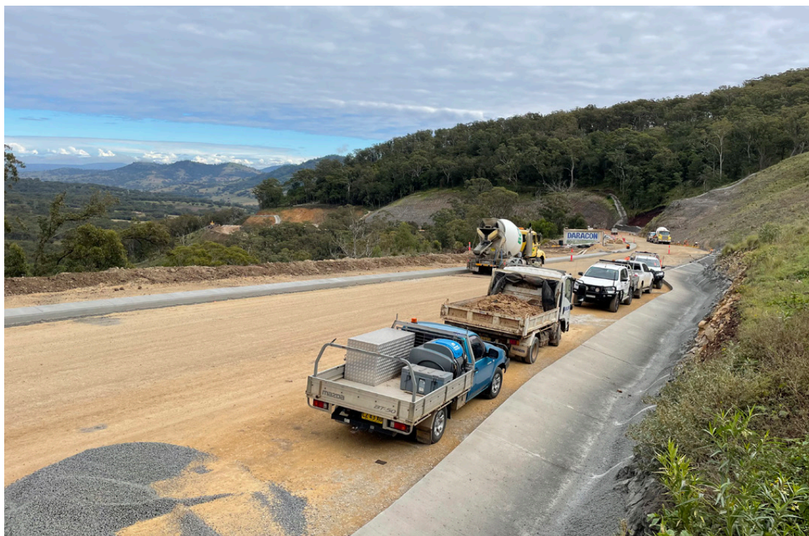
Concrete Kerbing
