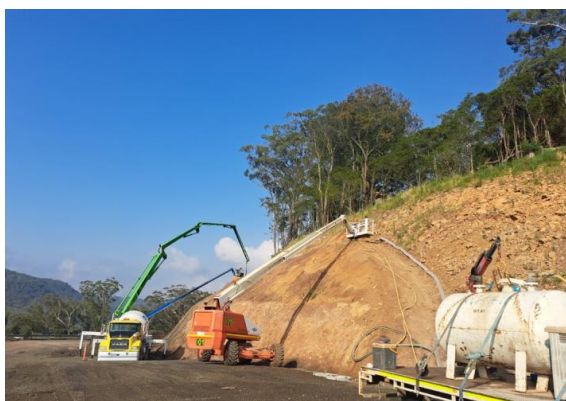
Catch Drain Construction
