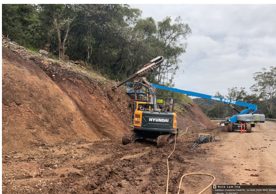
Rock Bolt Drilling
