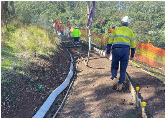
Catch Drain Construction
