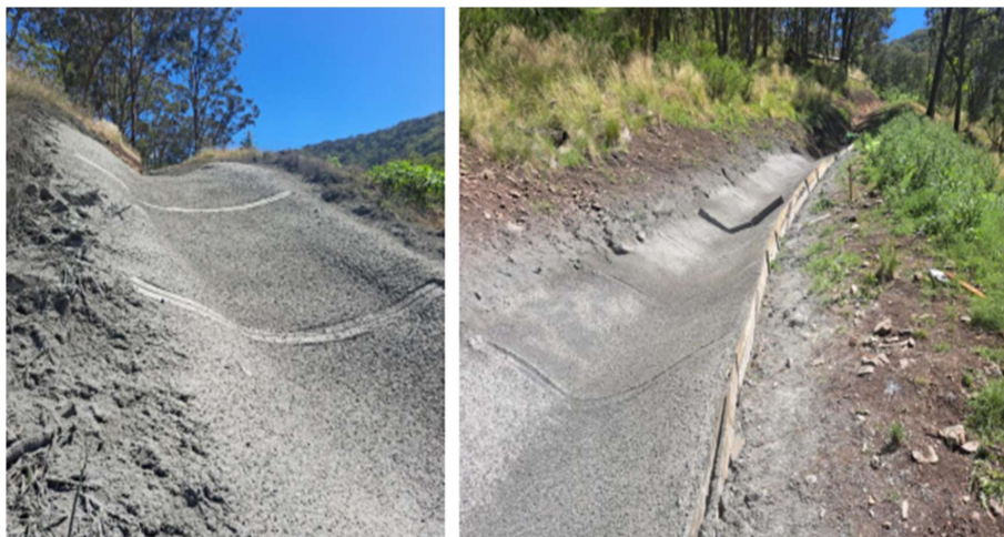
Shotcrete Drain and Batter Chute
