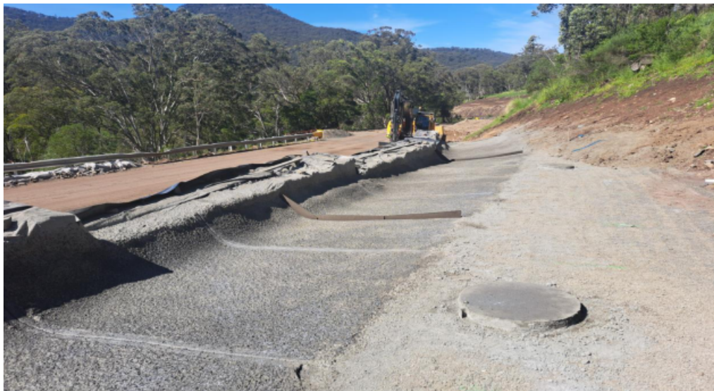
Shotcreting MT10 Catch Drain
