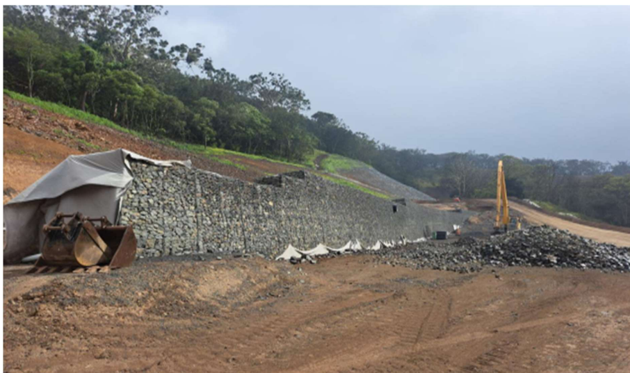
Gabion Wall Construction – Section 3
