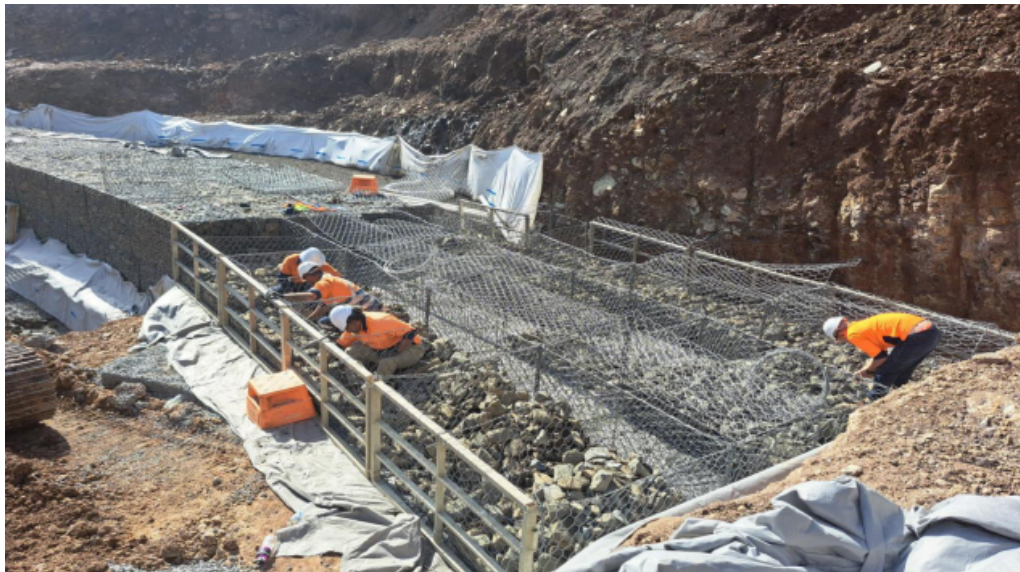
MT 40 Gabion Wall Construction Layer 3
