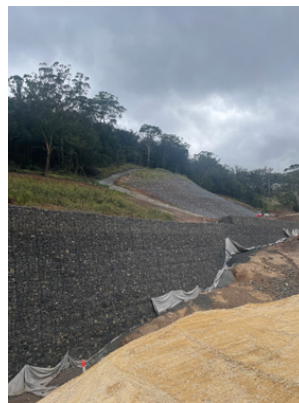
Section 3 Gabion Wall construction
