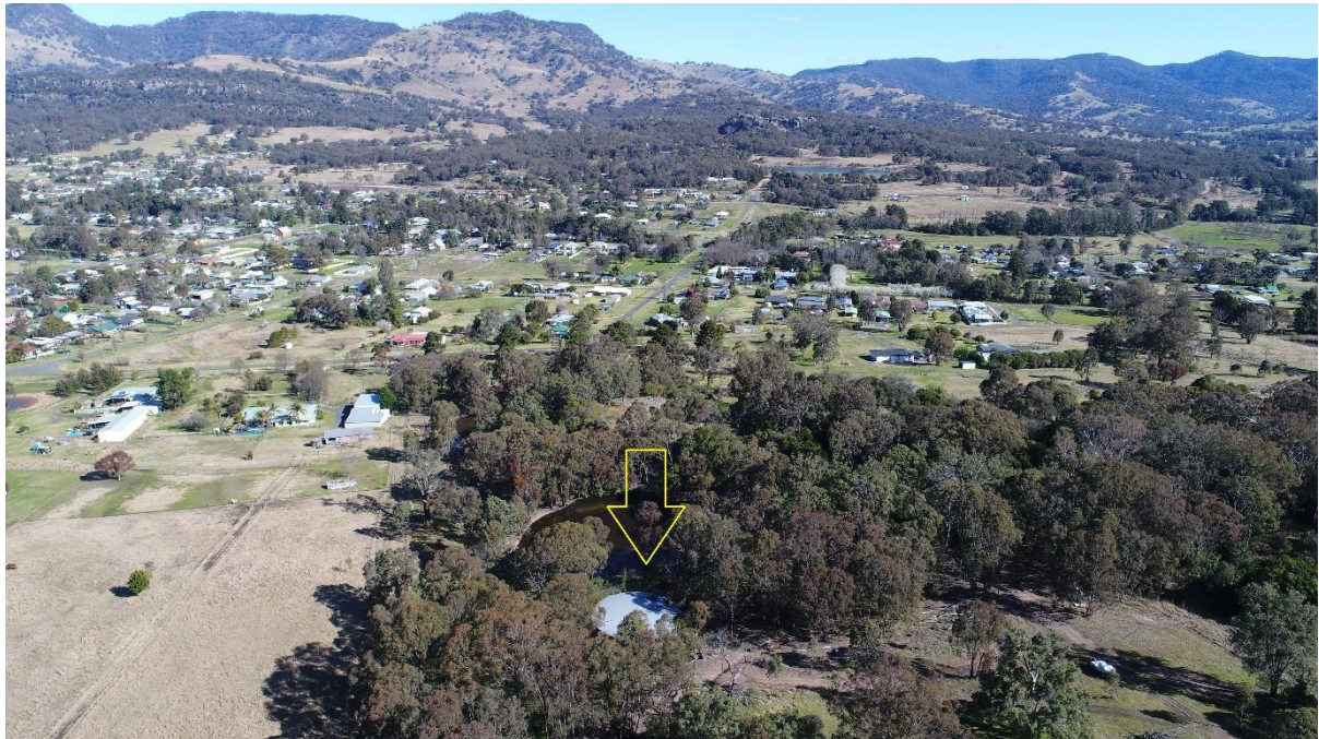
Doughboy Street Redundant Tank (looking south to Murrurundi)
