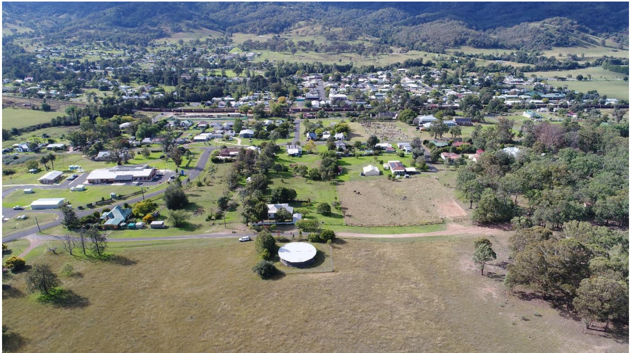
Paradise Lane Reservoir looking north to Murrurundi
