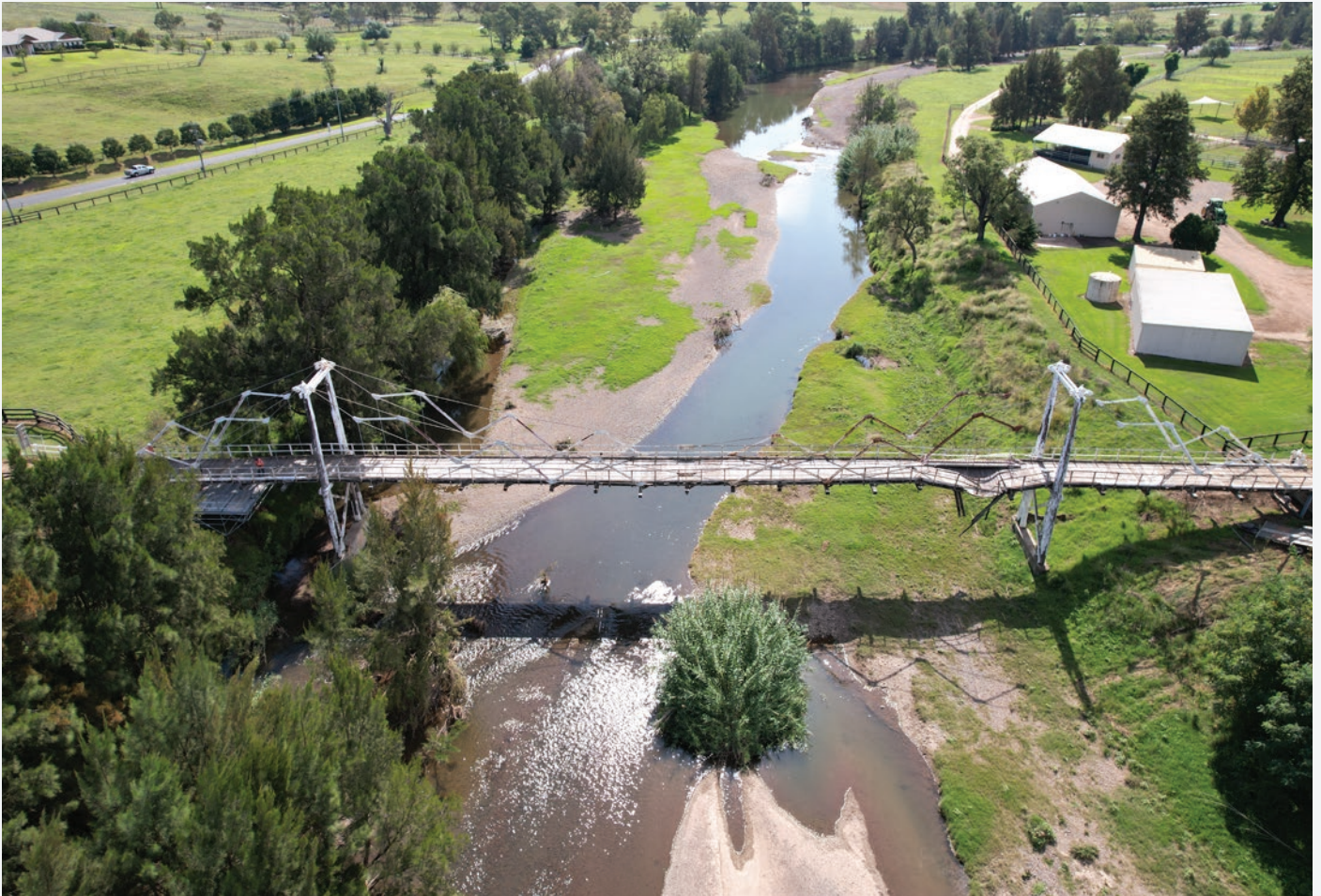
Allan Bridge before restoration
