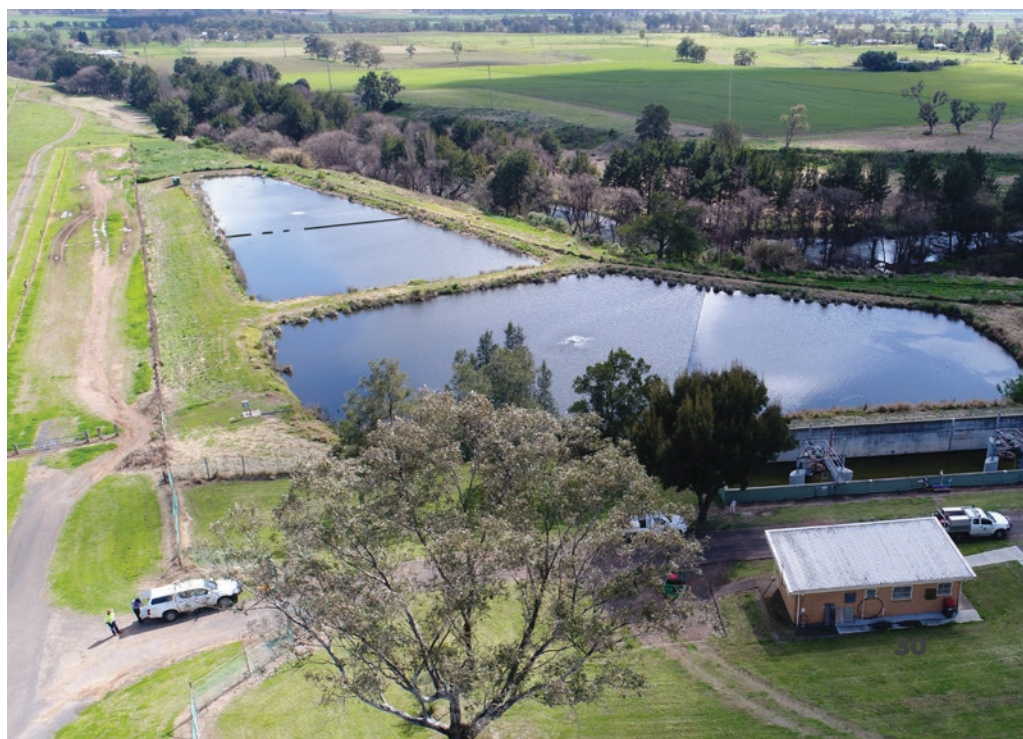
Aberdeen Sewer Treatment Plant
