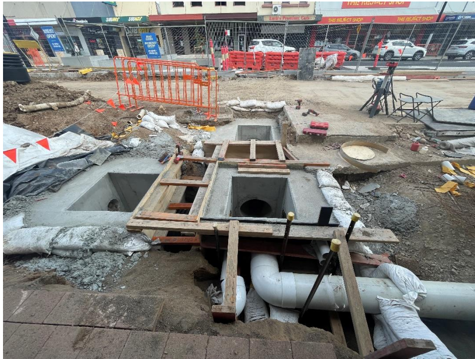
Image 10 – Storm Water Pit Construction
