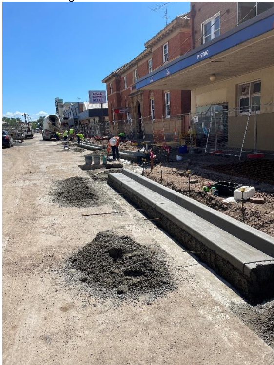
Image 5 – Construction of Kerb
