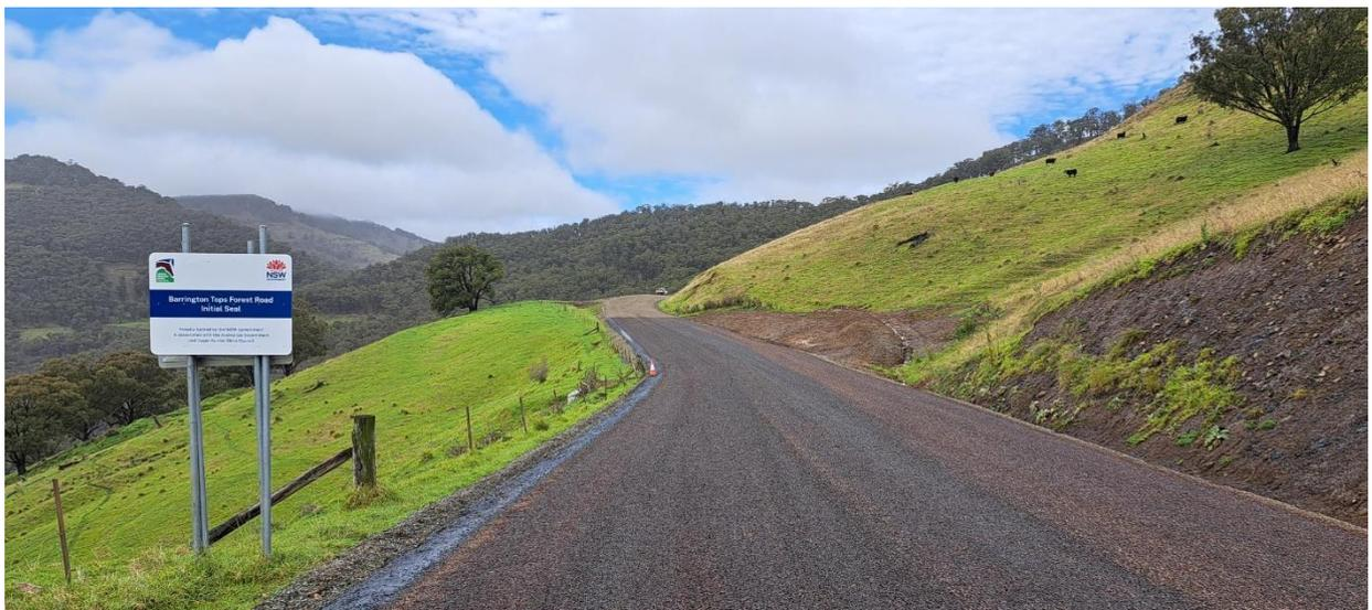
Figure 1: Barrington Tops Forest Road – two-coat seal completed to Ch 6,600
