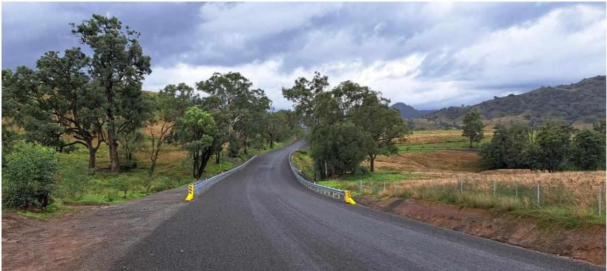
Figure 3: Hunter Road – sealed with guard rail at Ch 2,700
