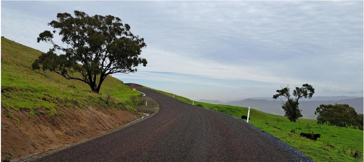
Figure 2: Barrington Tops Forest Road – two-coat seal at Ch 6,300
