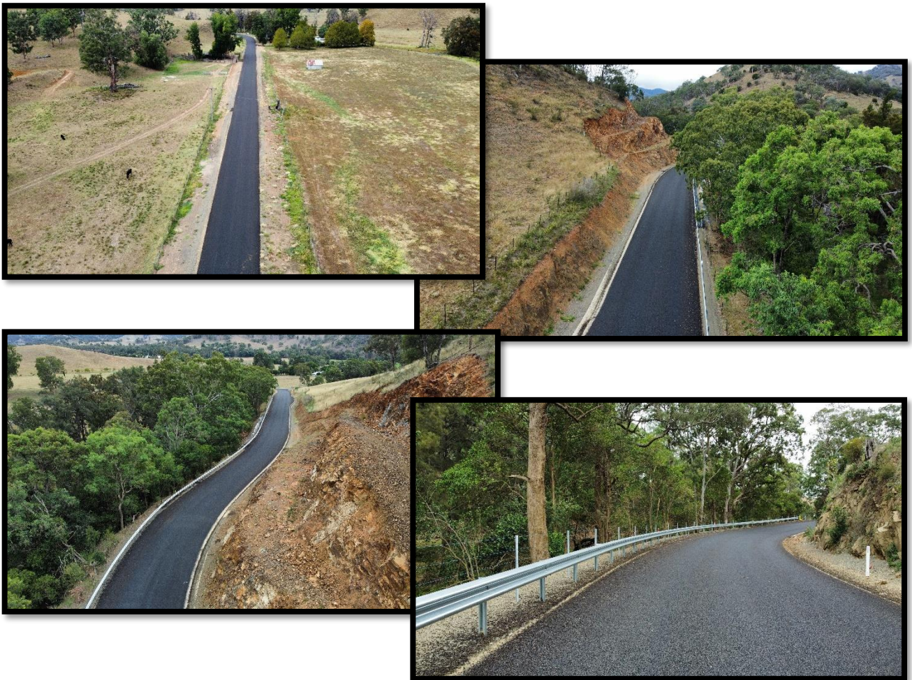
Drone photos of Moonan Brook Road Project
