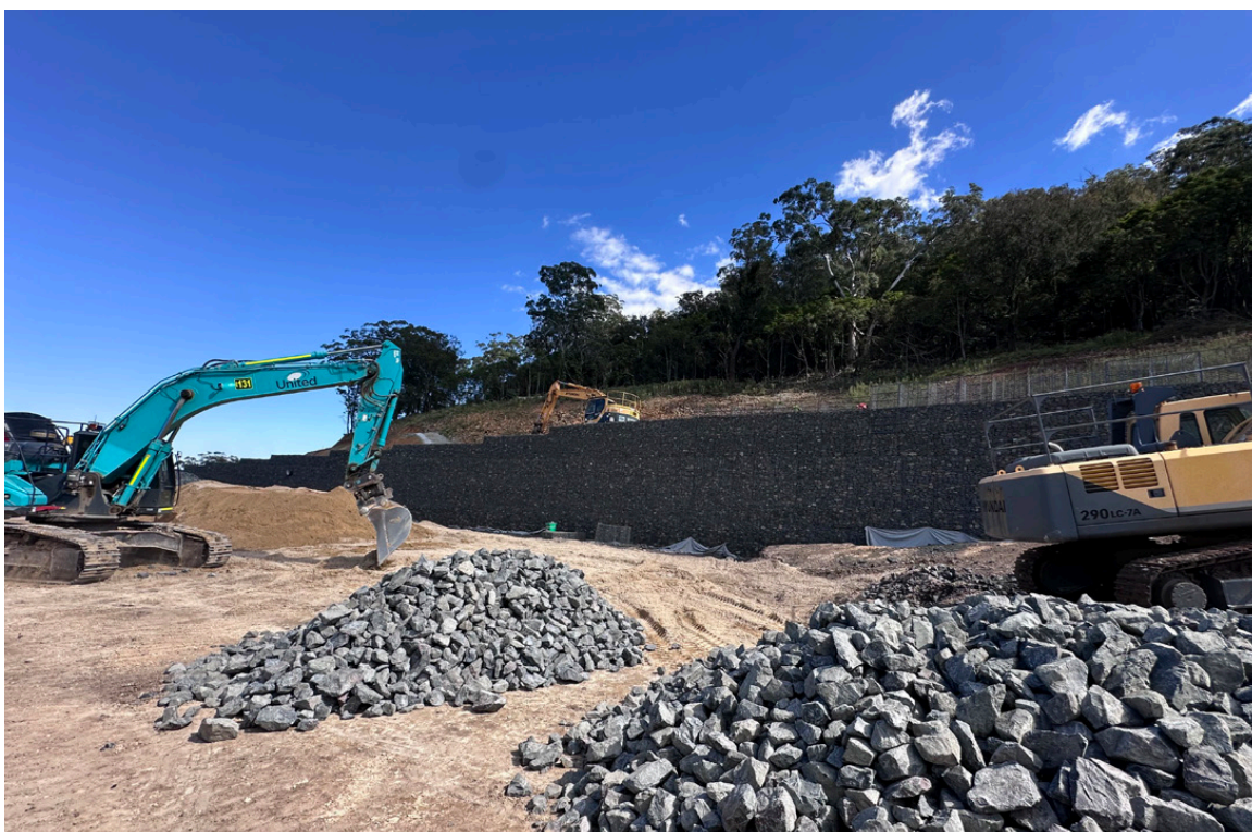
Completed Gabion Wall
