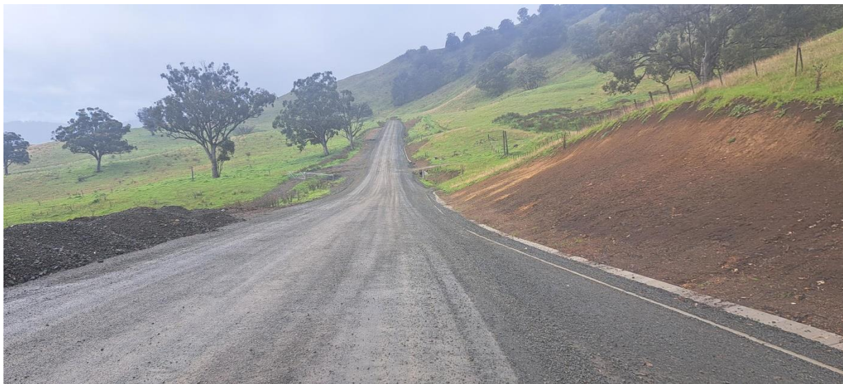
Figure 2: Barrington Tops Forest Road – completed pavement ready to be sealed at Ch 5,500
