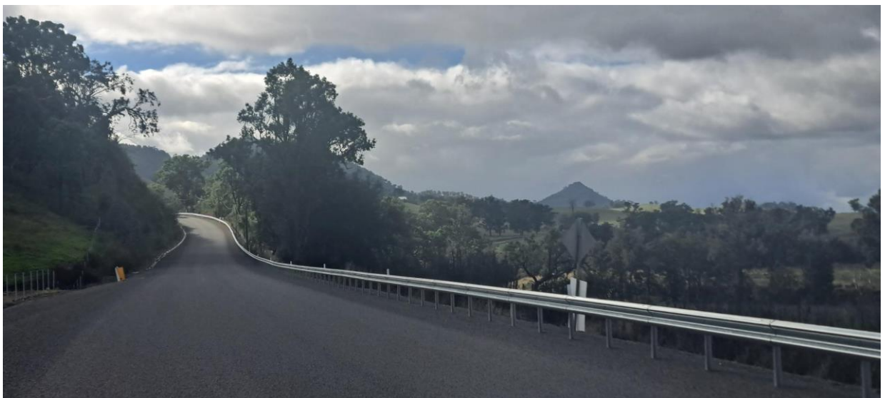
Figure 4: Hunter Road – sealed with guard rail at Ch 600
