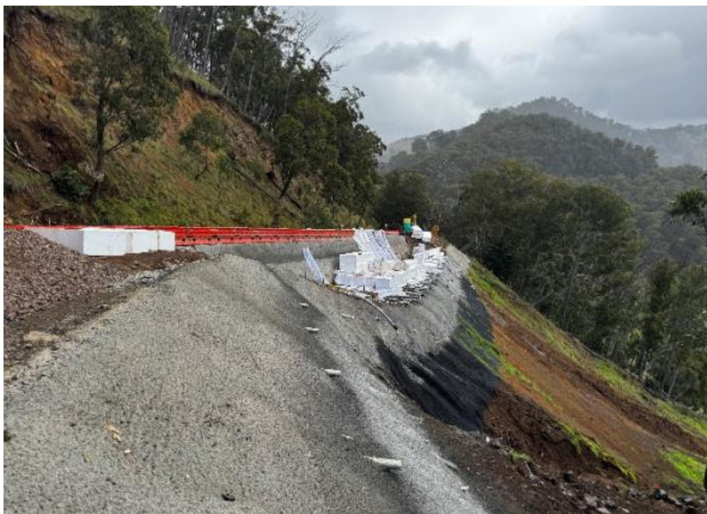
Figure 1: Landslip remediation works at BTF Road at Ch. 8200
