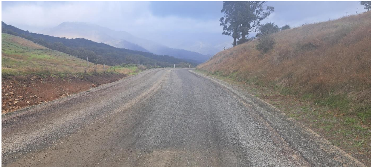
Figure 1: Barrington Tops Forest Road – two-coat seal completed to Ch 5,200
