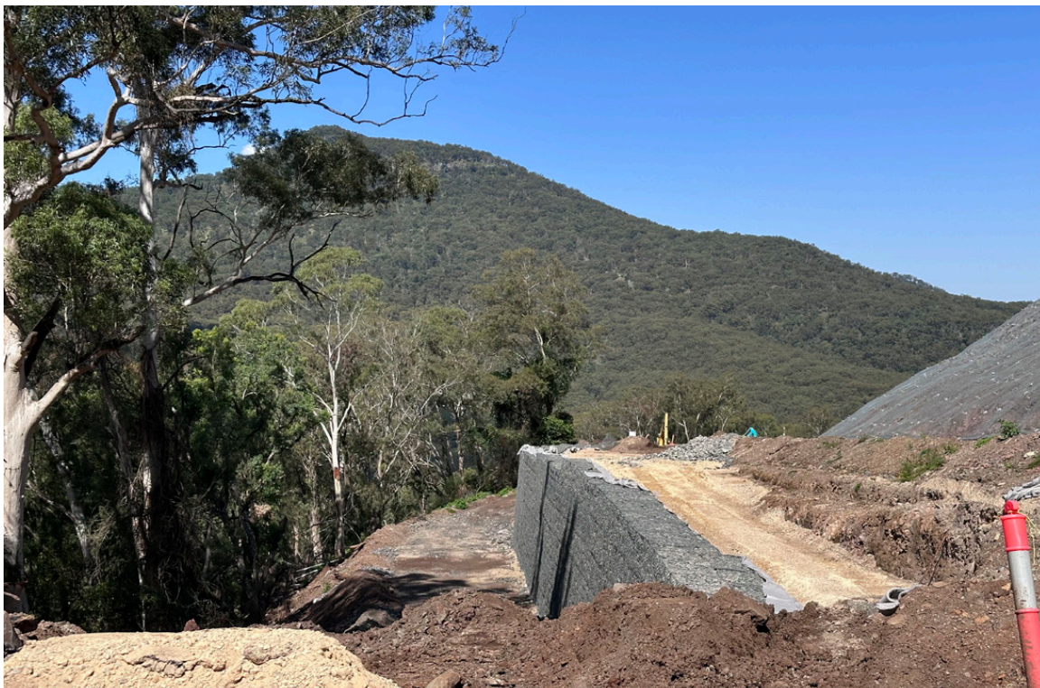
Completed Gabion Wall
